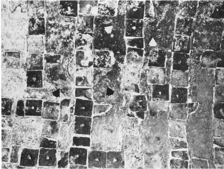
Fig. 22. Detail of remains of brick lining on intrados of N.II.1 showing holes in bessales. Arrows indicate impressions of brick stamps where the bipedales have fallen away.
