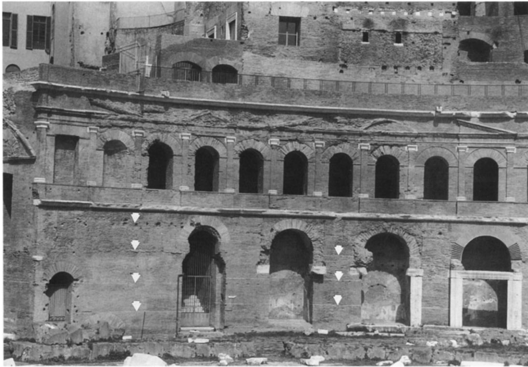
Fig. 3. View of Hemicycle elevation at north end. Arrows indicate courses of bipedales.
