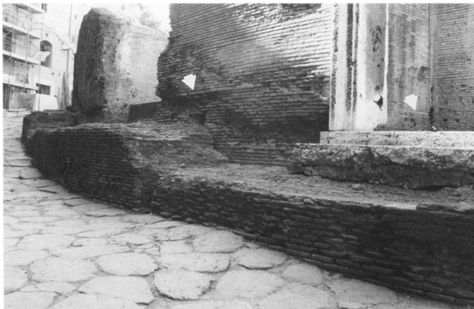
Fig. 15. View of rooms along Via Biberatica showing courses of bipedales (indicated with arrows) marking floor levels of H.II.5 and H.III.6
