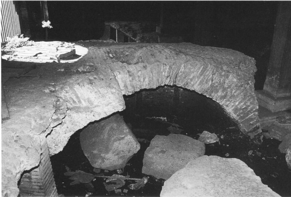
Fig. 3. Photo of the remains of the bipedalis ribbing in the substructure vault of the north portico of the Column courtyard. The opus caementicium drain wall is visible in the background under the vault.
