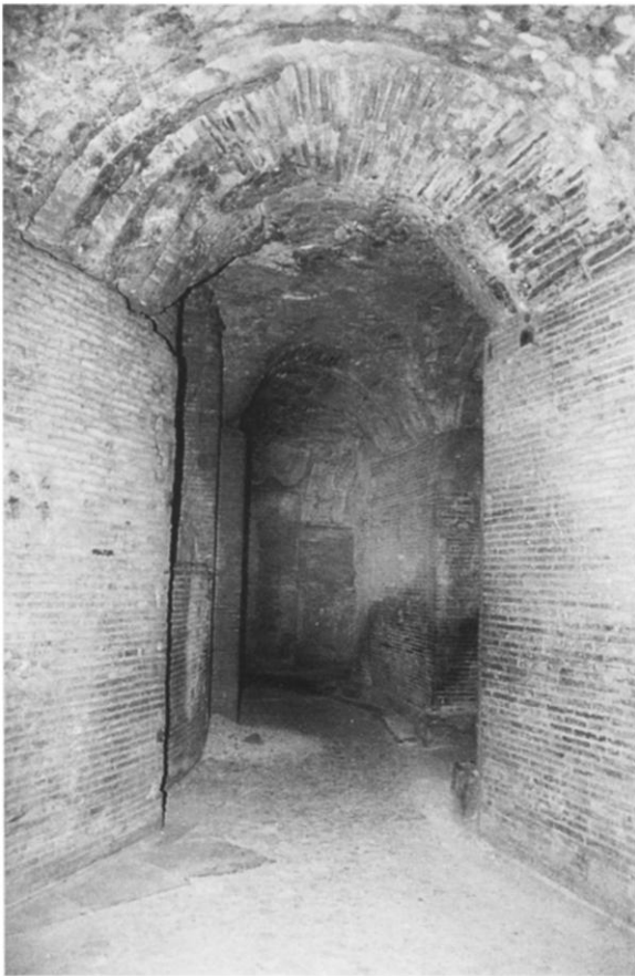
Fig. 11. Brick vaulting ribs in North Wing corridor outside of room N.II.6
