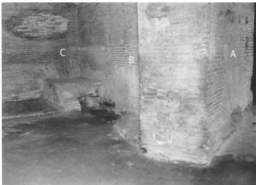
Fig. 4. View of room N.II.4 showing concrete drainage channel surrounded by relieving arches (approximately same view as shown to the right of fig. 2). Arch B is built over the section of the channel that runs directly underneath the wall.
