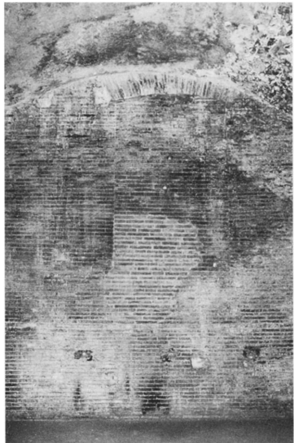
Fig. 15. Blocked opening in room H.II.4
