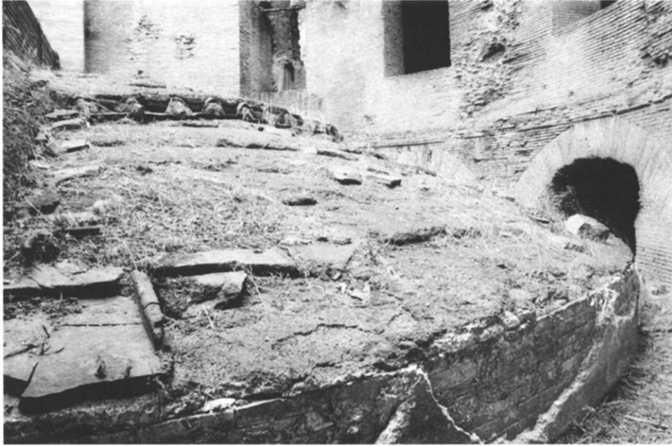
Fig. 12. Extrados of N.Ap showing remaining roof tiles on semidome
