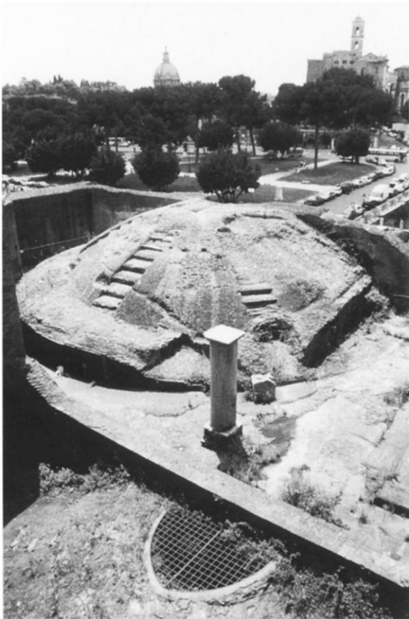
Fig. 13. Overview of extrados of H.ApN showing stairs and cut away portion of vault to right
