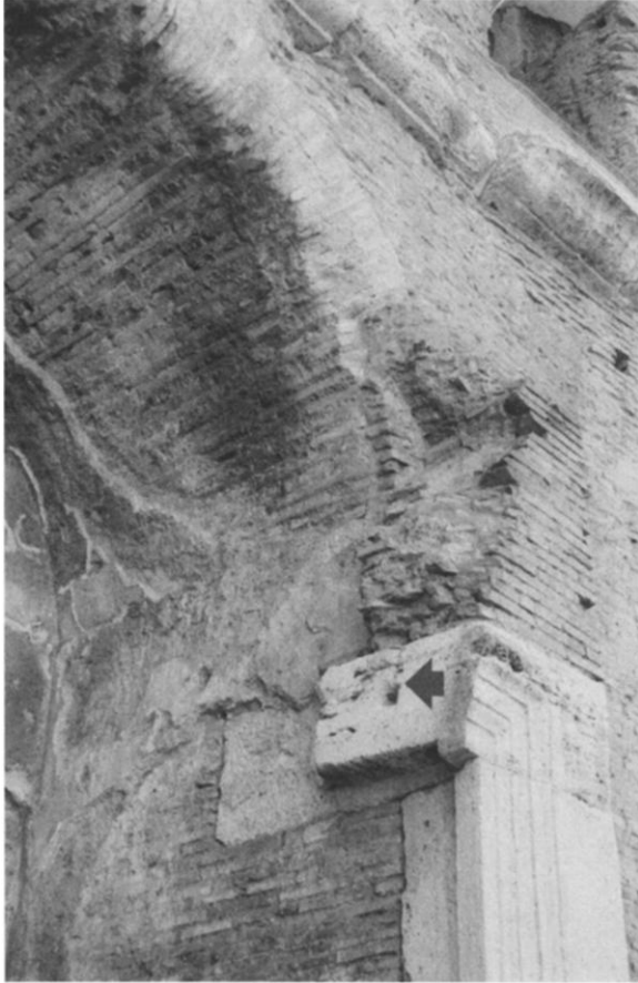
Fig. 18. Detail of corner block of travertine lintel of room at H.I.8 with dowel hole and pour channel (indicated by arrow). Note the bipedalis ribbing of the vault.
