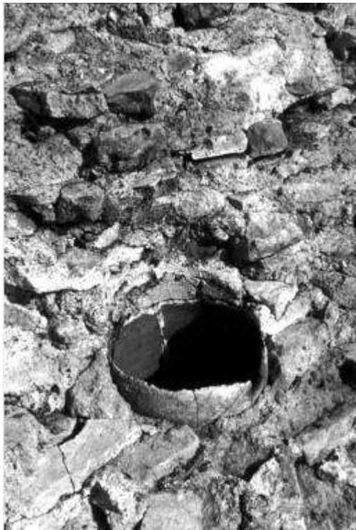
Figure 10. Remains of a series of vertical terracotta tubes, diameter cm 25, h preserved cm. 250, buried in the remains of the vault. Above the ribbed sections of the vault, the weight of the concrete was adapted to need using tuffo giallo and gray pumice.
