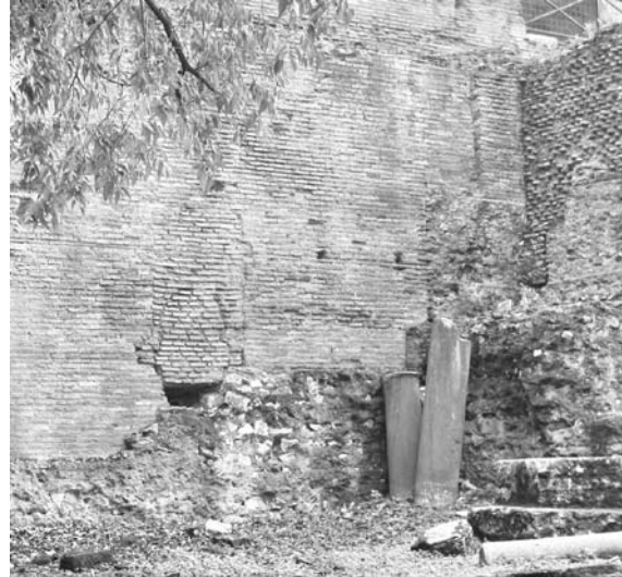
Fig. 15a-c: Pronaos, south-east end. The construction of the projecting pronaos was prepared building a foundation, in part against the ground and in part against blocks, and then an elevated section with blocks at each end. Both were clearly bonded to the foundation and the perimeter wall of the Basilica; consequently it must be attributed to the first phase of the building, in Maxentius time.
