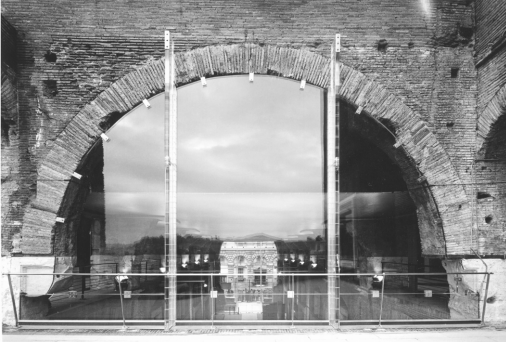
Figure 3. Closure in acrylic panels of the arch of the Great Hall facing Via Biberatica.
