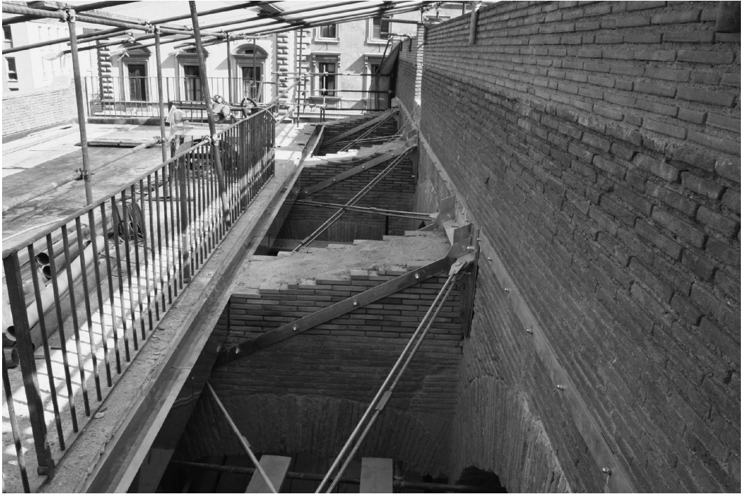
Figure 14. View of the southern lateral longer side of the Great Vault with the diagonally counterbraced shear reinforcements placed in the free spaces between the Vault itself and the Southern building, nearly the ending of the work.
