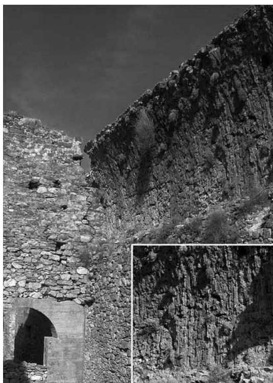
Fig. 16 Anamurium. Baths III 2 B. View of room G with inset showing detail of impressions in mortared fill of vault left by vertical bricks.
