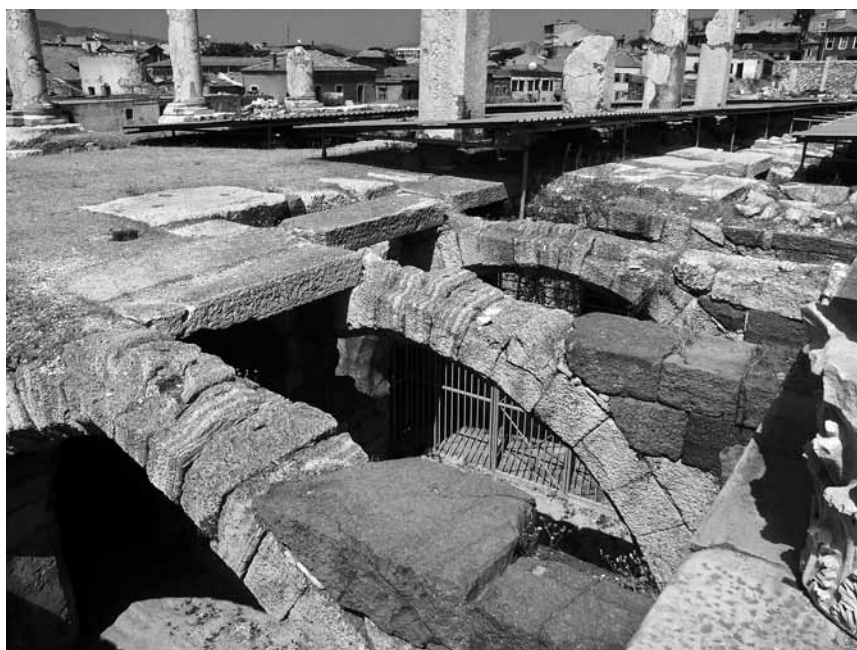
Fig. 11 Smyrna (modern Izmir). Basilica. View showing stone arches of substructure supporting flat slabs of flooring.
