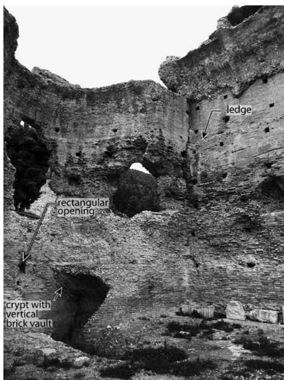
Fig. 4 Argos. Bath A. View into main hall A1 showing crypt and ledge that supported vertical brick vault.
