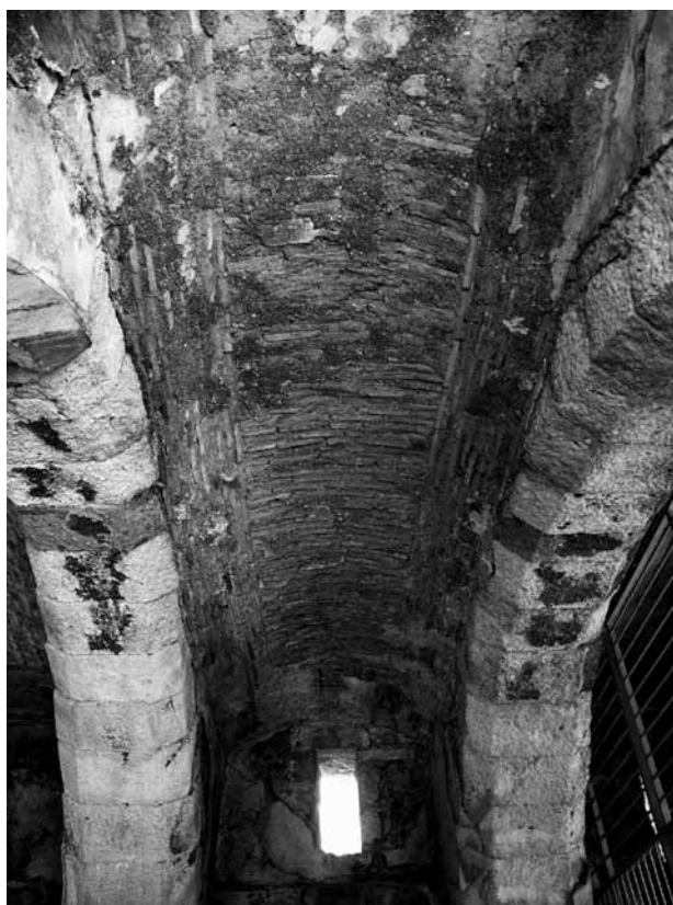
Fig. 12 Smyrna. Basilica. View shallow brick vault with vertical brick crown that replaced the stone slabs.
