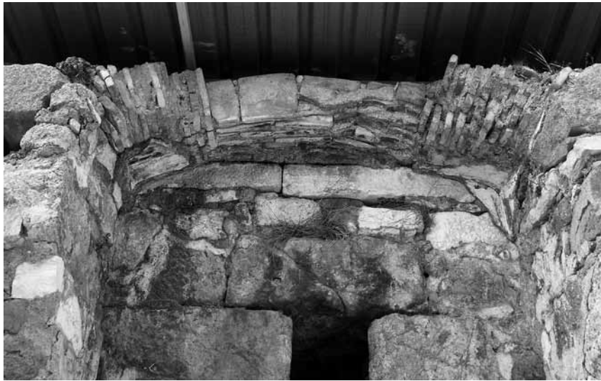
Fig. 13 Smyrna. Basilica. Detail of construction of partially fallen vault.
