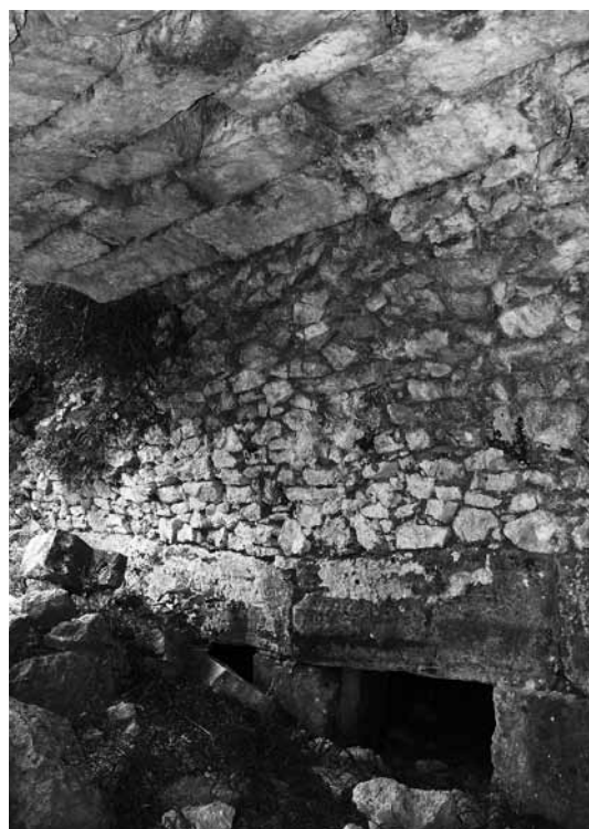
Fig. 17 Cremna. Agora Cistern. View of interior of one chamber showing the cut stone voussoirs at crown.
