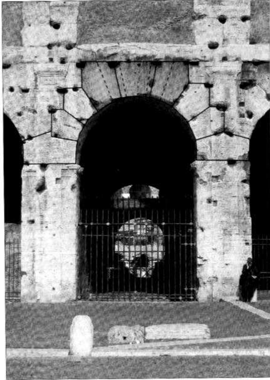
Fig. 23 Level I arch (bay 68) with nine voussoirs (outlined in solid black lines). The top three voussoirs (shaded) are substituted by five voussoirs (indicated with dashed lines) in arches with eleven voussoirs.
